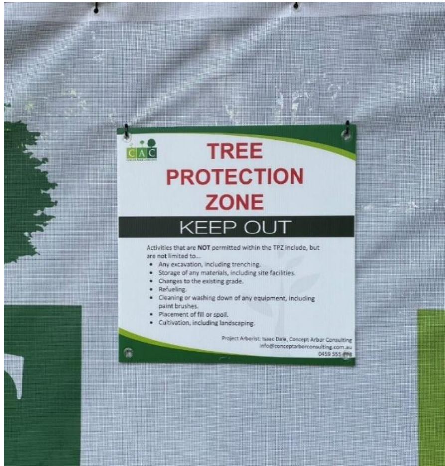
Figure B2: Example of a TPZ sign.
