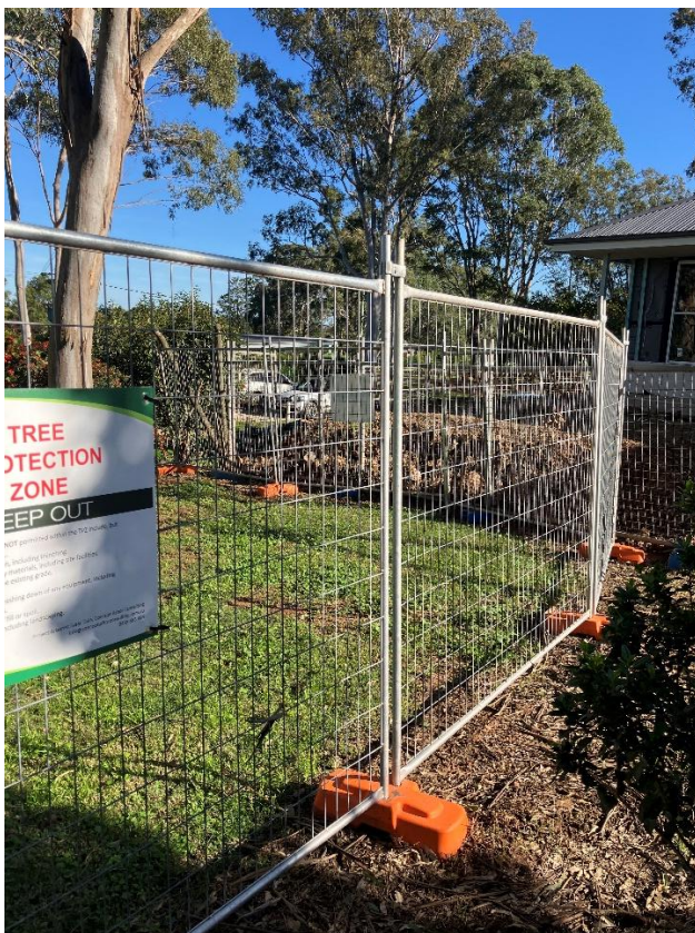
Figure B3: Example of rigid TPZ fencing.
