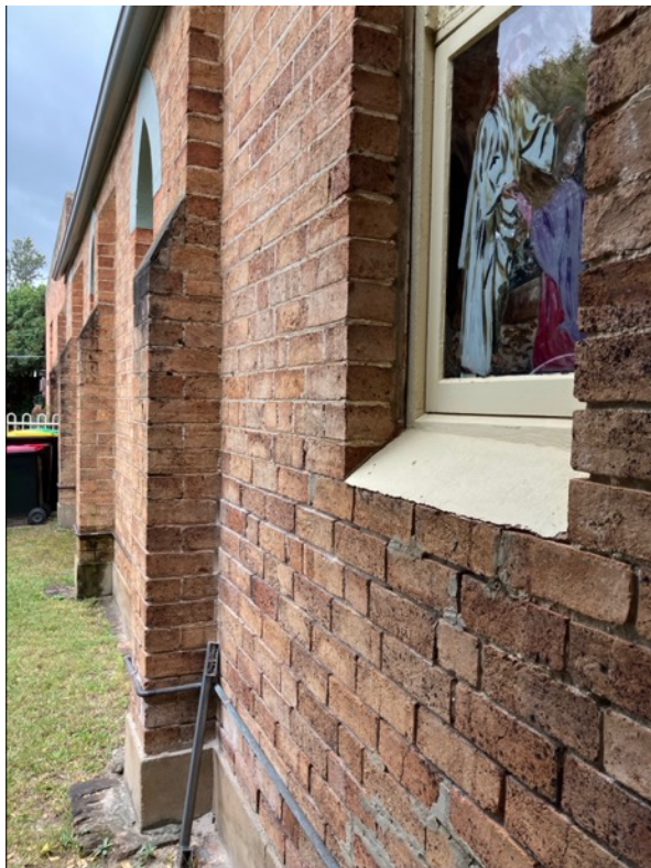
Figure 35: Buttresses to western elevation.
