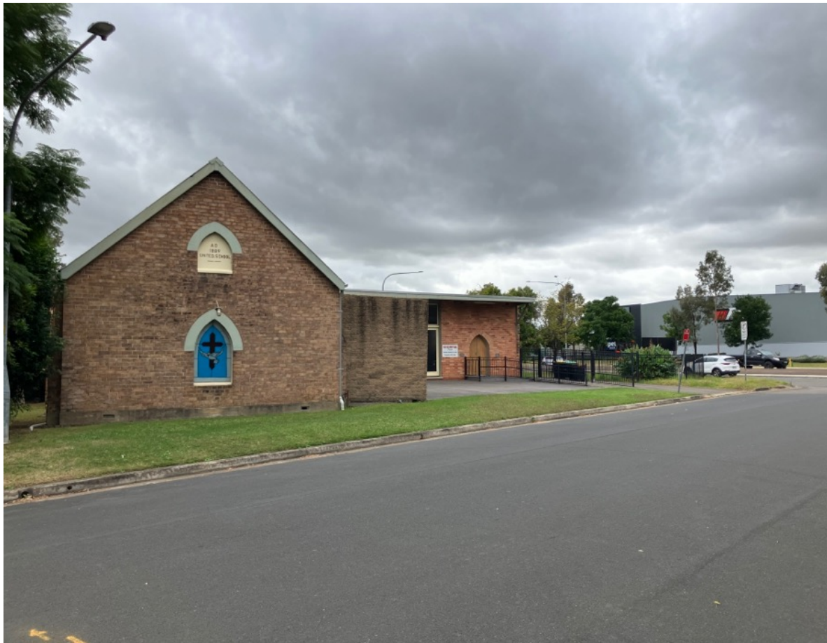
Figure 21: View to the church and Site from Stuart Street.
