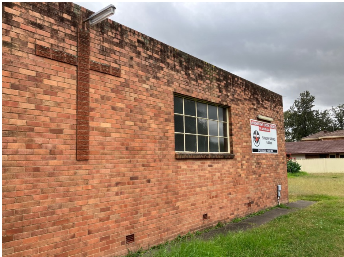
Figure 27: Presentation of eastern wall of the hall and classroom addition.
