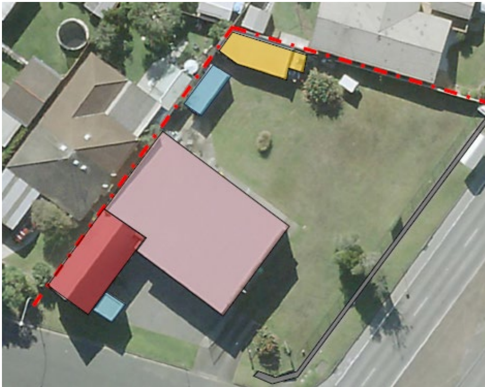
Figure 3: Aerial view of site showing various historical elements
