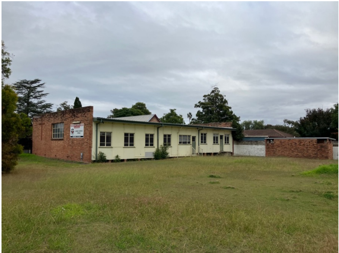
Figure 25: View towards the north elevation of the church hall and classroom
