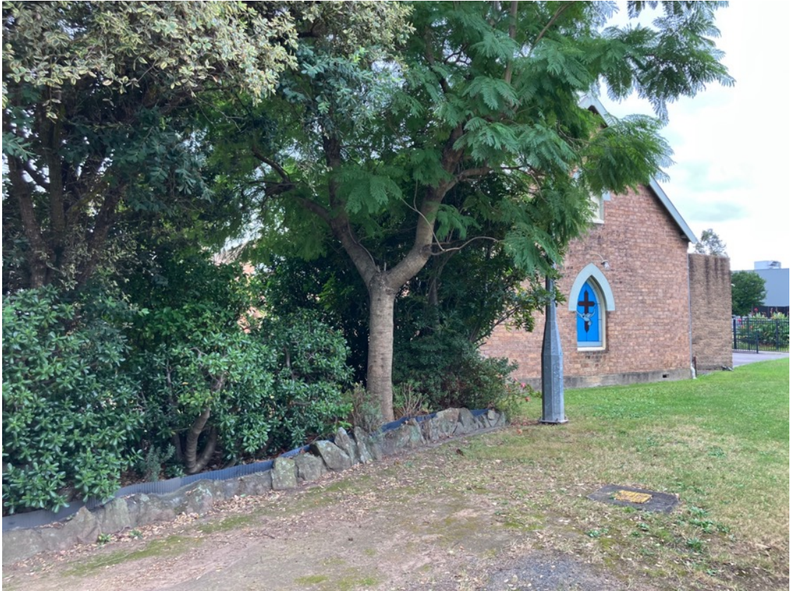
Figure 22: View to the front of the church from the adjacent property on Stuart Street.
