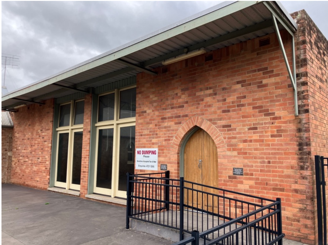
Figure 28: Presentation of the southern wall of the hall and classroom addition.
