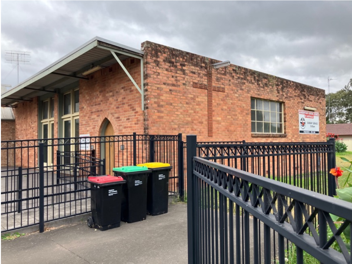
Figure 30: View of the hall and classroom addition.
