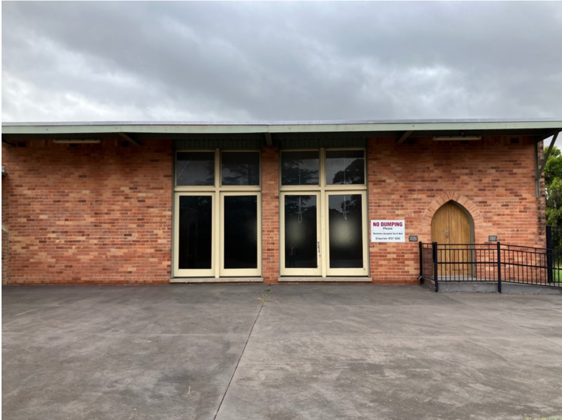
Figure 32: Concrete forecourt and southern elevation of the hall and classroom addition.
