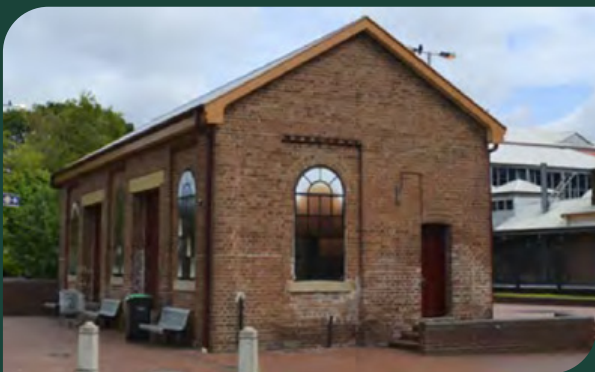
Figure 7 – Heritage goods shed outside the train station (St Marys Town Centre Structure Plan)
