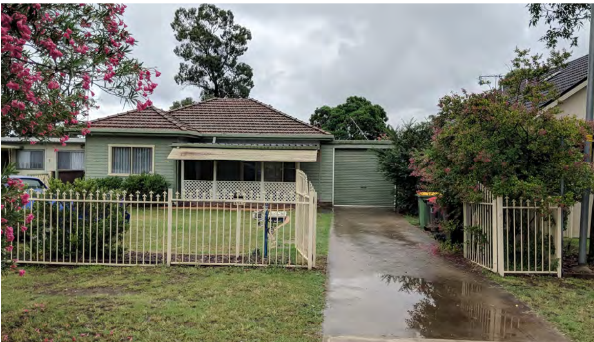
Figure 28 – Example of an older detached dwelling in Penrith
