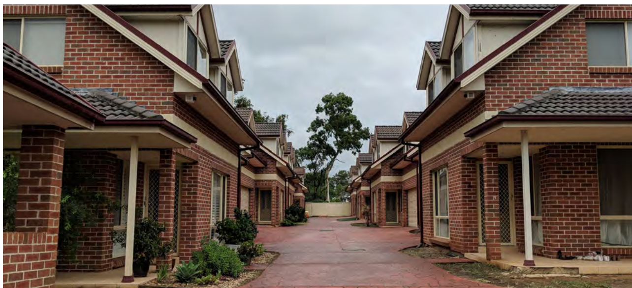
Figure 31 – An example of existing medium density housing in Penrith
