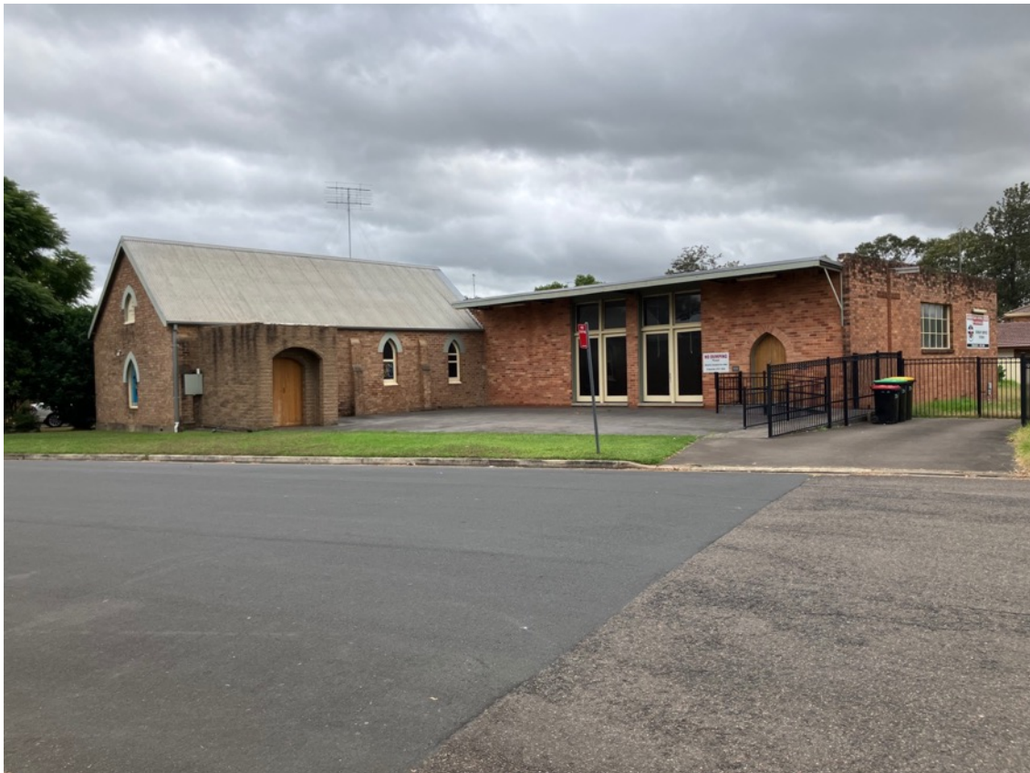
Figure 23: View to the Church and hall and classroom extension from Stuart Street.
