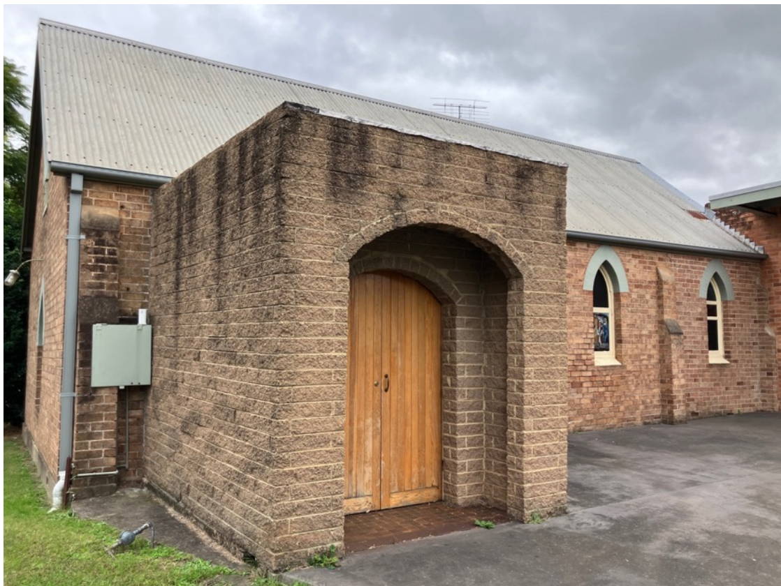
Figure 33: Non-original c.1970s narthex addition to the church.
