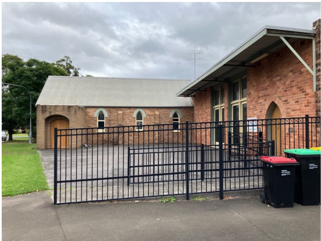
Figure 31: Eastern elevation of the church and southern elevation of the hall and classroom addition.
