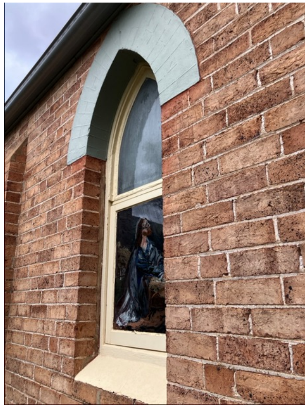
Figure 36: Windows to western elevation.
