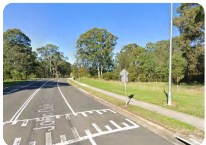
Figure 55. John Oxley Avenue (Google Streetview 2025)
