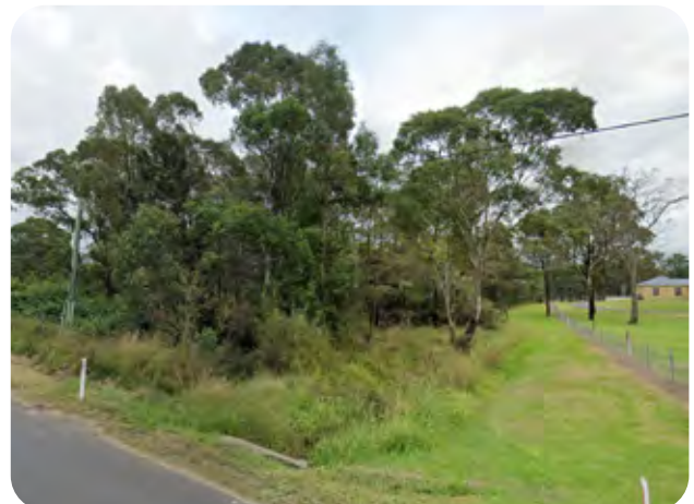
Figure 52. Tempest Street (Google Streetview 2021)
