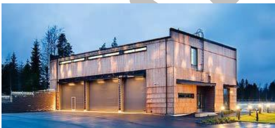
Figure 64: Centralised collection station servicing multiple developments/stages
