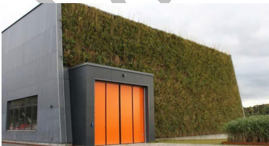
Figure 65: Centralised collection station servicing multiple developments/stages
